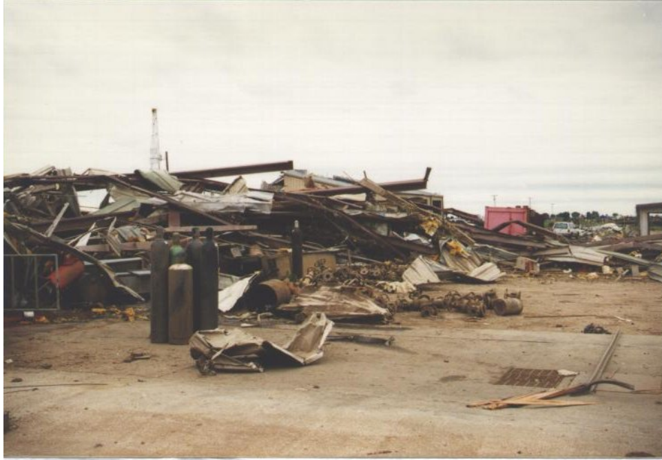
MBS: DOD 8: Total destruction of building
