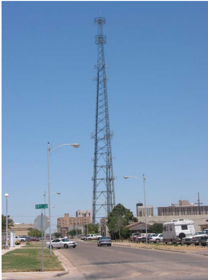
FST: Free-standing Truss Tower
