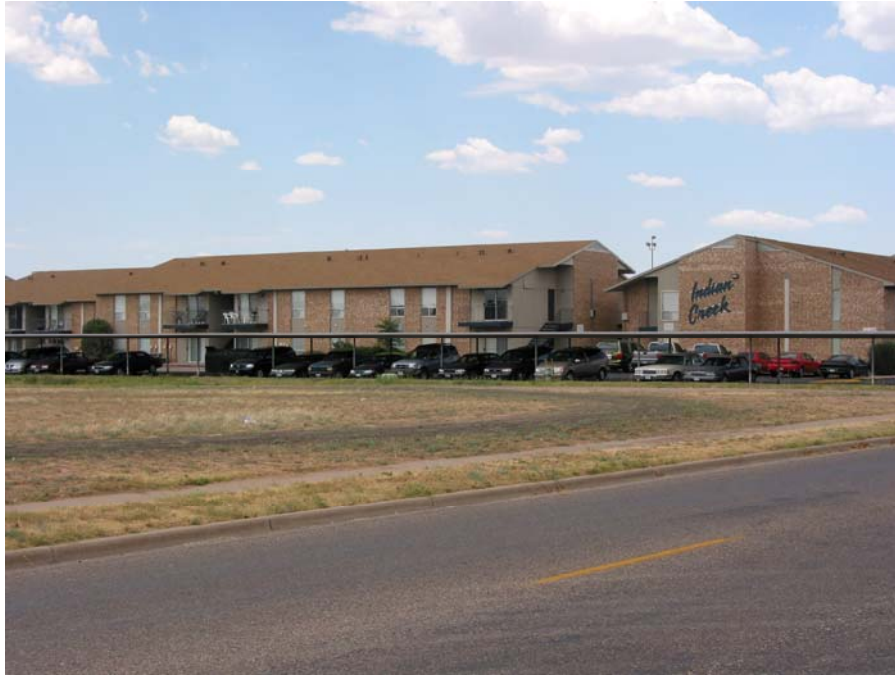
ACT: Gable roof, asphalt shingles, wood decking, light-framed, wood construction, brick veneer, wood stud walls, balconies
