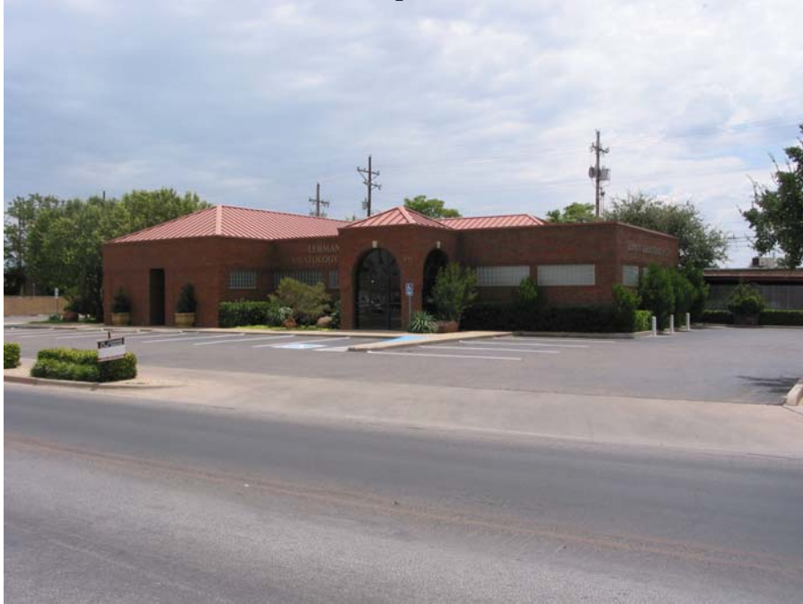
SPB: Hip roof, metal panel roofing, Light-frame steel construction, metal stud walls, brick veneer
